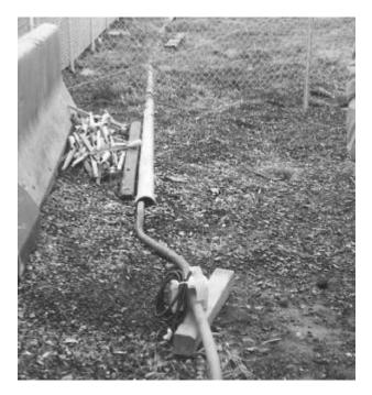
Figure 5-18. Example of encapulated abovesurface heat-trace lines entering sub-surface location around the perimeter of a HTRW site encapsulated heat-trace lines to provide additional protection from heavy truck traffic. These would be the only areas where truck traffic would be allowed to enter or exit from the site. Figure 5-18 illustrates encapsulated surface heat-trace line from entering subsurface location at the entrance of a HTRW site.
