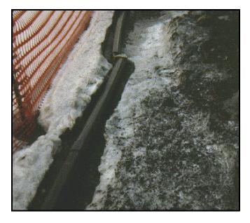
Figure 5-17. Example of encapulated heat-trace line in PVC conduit around the perimeter of a HTRW site
